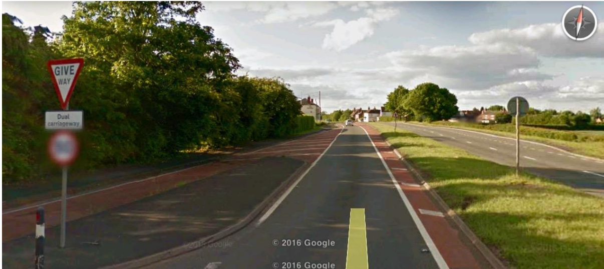
Photograph 6: The image shows a section of the A449 at Ombersley, Worcestershire (looking north). It has had its speed limit lowered and the road has been reduced in size from two lanes to one by Worcestershire County Council.
